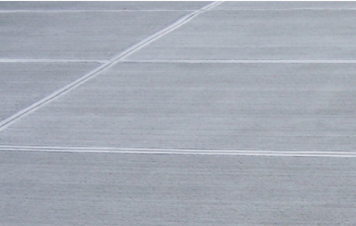
P2 Podium pavement Insitu concrete - Stadnard grey
