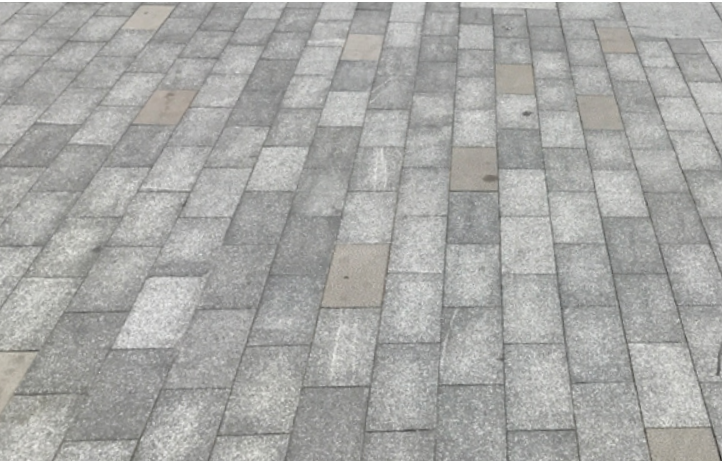
P4 Small format pavement 400x200x50mm concrete unit paving. Supplier: Stonevue - Hawthorne
