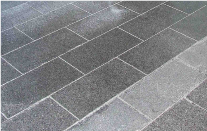
P1 Civic pavement 800x300x50mm concrete unit paving. Supplier: Stonevue - Hawthorne
